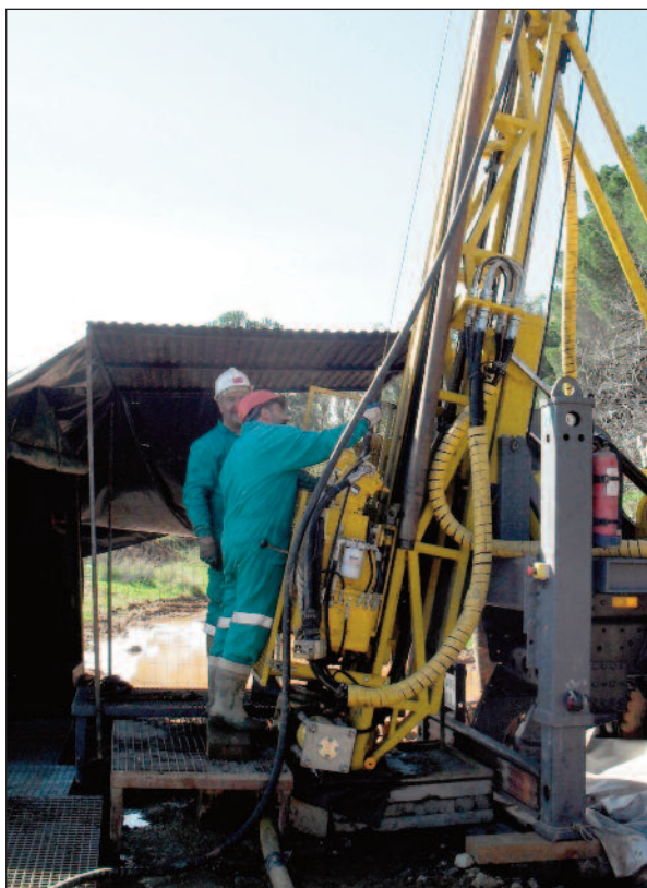
Joint Venture drilling operations at La Zarza, March 2010.
