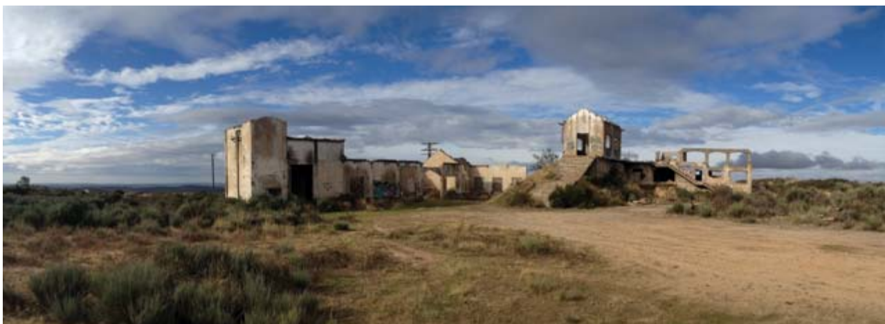
View of old mine buildings at Barruecopardo
