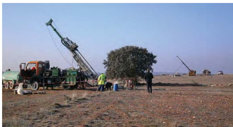
Two drill rigs operating on El Facho structure, Zamora
